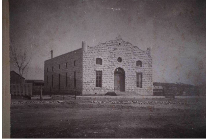
The Halle under construction 1899
